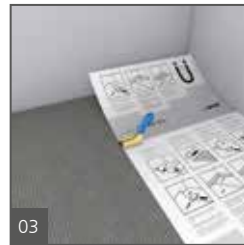
03 Insert wedi Subliner Dry with the printed side facing upward and press on with a rubber roller or wooden float. Remove airpockets and other foreign particles from below the sheets.
