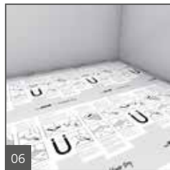
06 In complete wet rooms, wedi recommends to flash Subliner Dry up the wall by 2" (50.8 mm) where it is still invisible behind baseboard tile or wood applications.
