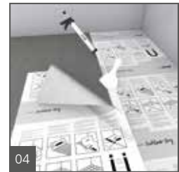
04 The sheets must overlap 2" (50.8 mm) at joints/transitions. Leave these overlapping areas free of any thinset and use tape to keep them folded upward and/or clean. Once the thinset has cured, apply wedi Sealant 620 as a full bed onto the lower mat's seam connection area and press the top overlap flat into the wedi Sealant 620.
