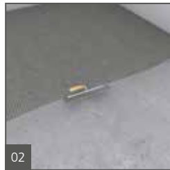
02 Apply thinset mortar to the prepared subfloor using a 1/8 x 1/8" (3.2 x 3.2 mm) or 1/4 x 1/4" (6.4 x 6.4 mm) notch trowel.
