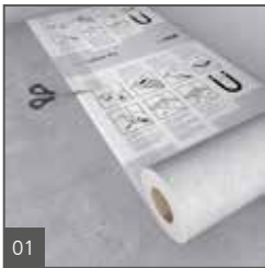
01 Lay out wedi Subliner Dry and cut to size using a knife or scissors.
